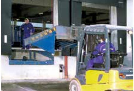
Remove old dock leveller, adjust pit if necessary (e.g. with fitting plates or support brackets)
