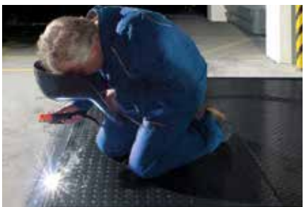
Weld to the edge brackets – done!
